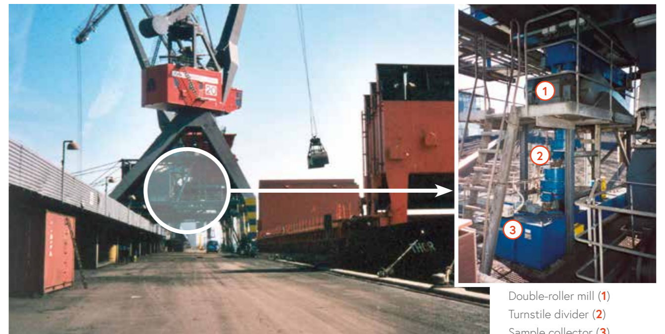
Sampling in coal unloading crane
